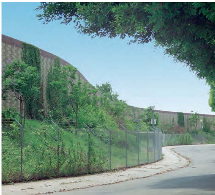
Figure 6 – Landscaped Earthen and Concrete Sound Barrier (above)/ Source: D. Chan, personal communication, December 7, 2011
